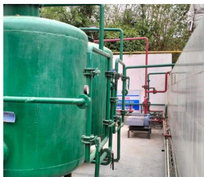
STP installed (250 KLD)
