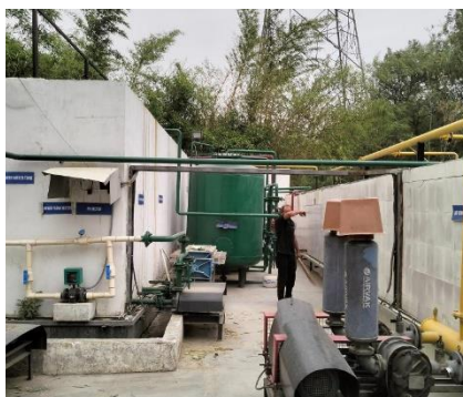
STP installed (250 KLD)
